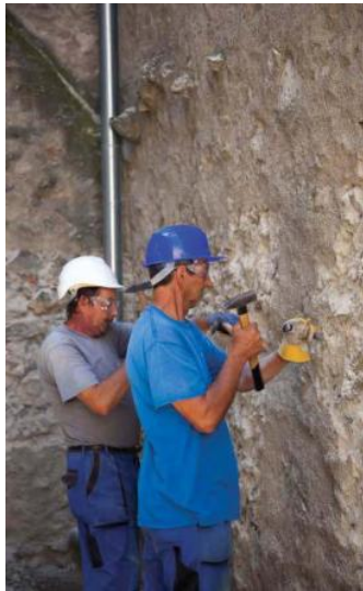
Exhausting removal of the cement mortar (Ižvolt and Smatanová 2014)
