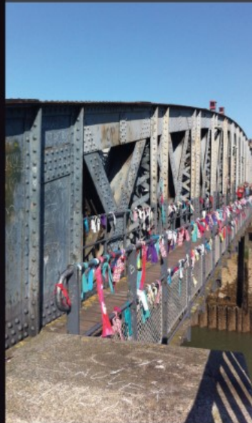
Colbert Swing Bridge in Dieppe Normandy - FRANCE
